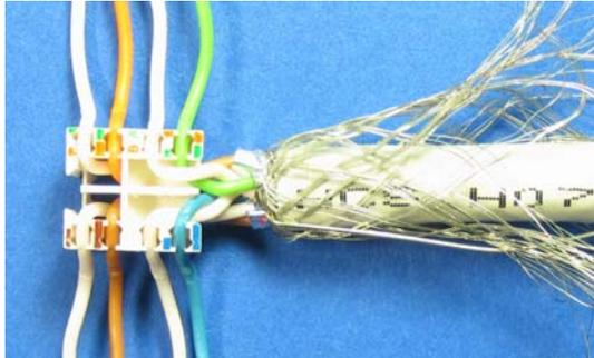
**5** Cut the wires flush with a sharp tool.
