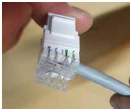
Place cap on jack and press to make sure it is fully seated The cap opening allows the cable to move from side to rear
