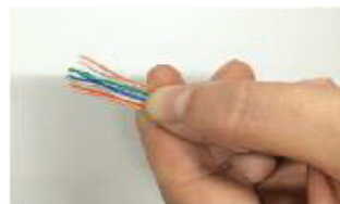
Step 3: Arrange the pairs according to desired wire-map
